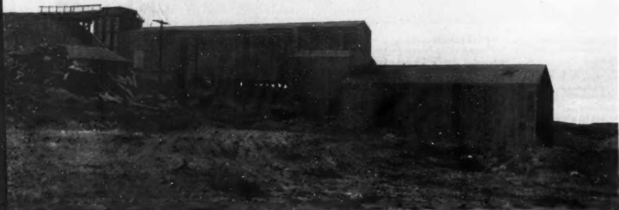
The new 100-ton-per-day sulphur flotation mill of the Wyoming-Gulf Sulphur Corporation was built in six months and has been in successful operation since November.
